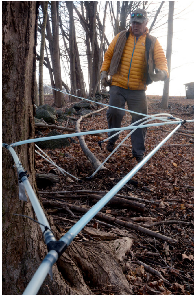
Here and below: Jahoda works on laying taplines at the Red House location on Chapelle Road in Lebanon
